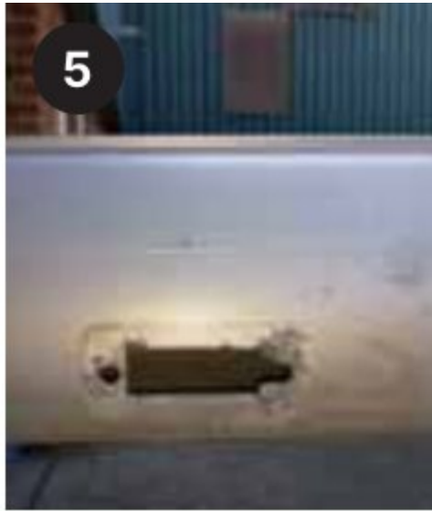
Picture 5: corrosion around the lower rivet hole at the spinnaker halyard exit
