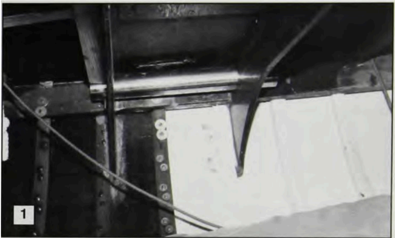
Photo 1 (Windermere class rig): the stainless steel tube positioned under the deck.
